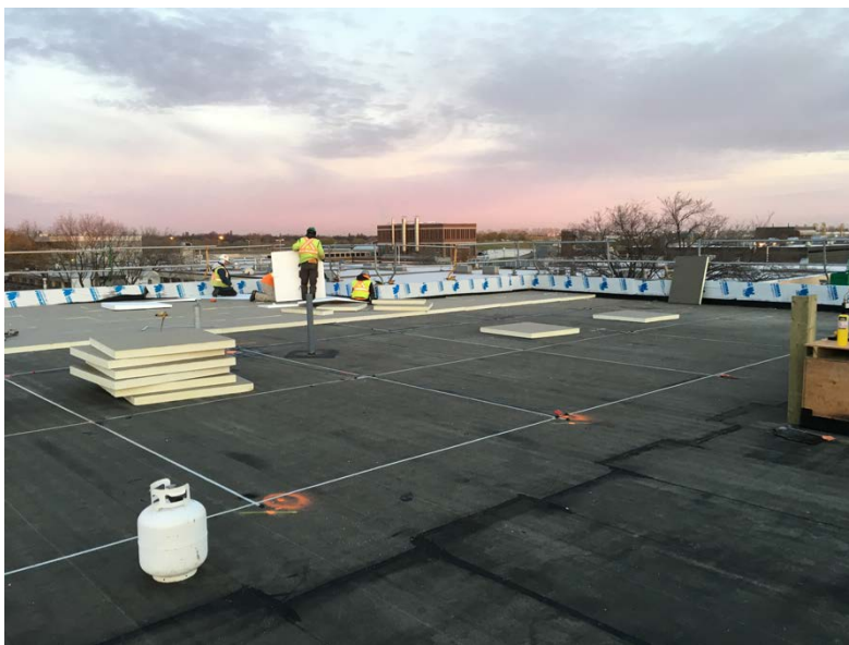
Figure 2. Sensor Grid Installation
